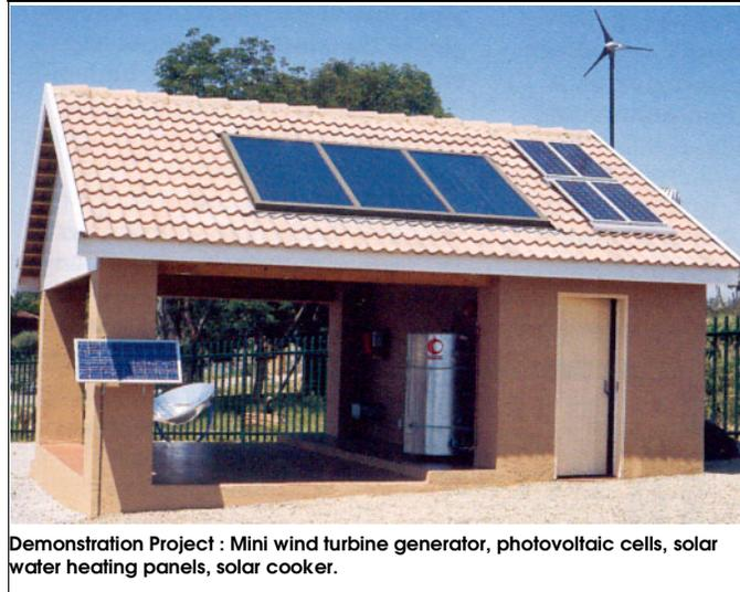
Demonstration Project : Mini wind turbine generator, photovoltaic cells, solar water heating panels, solar cooker.
